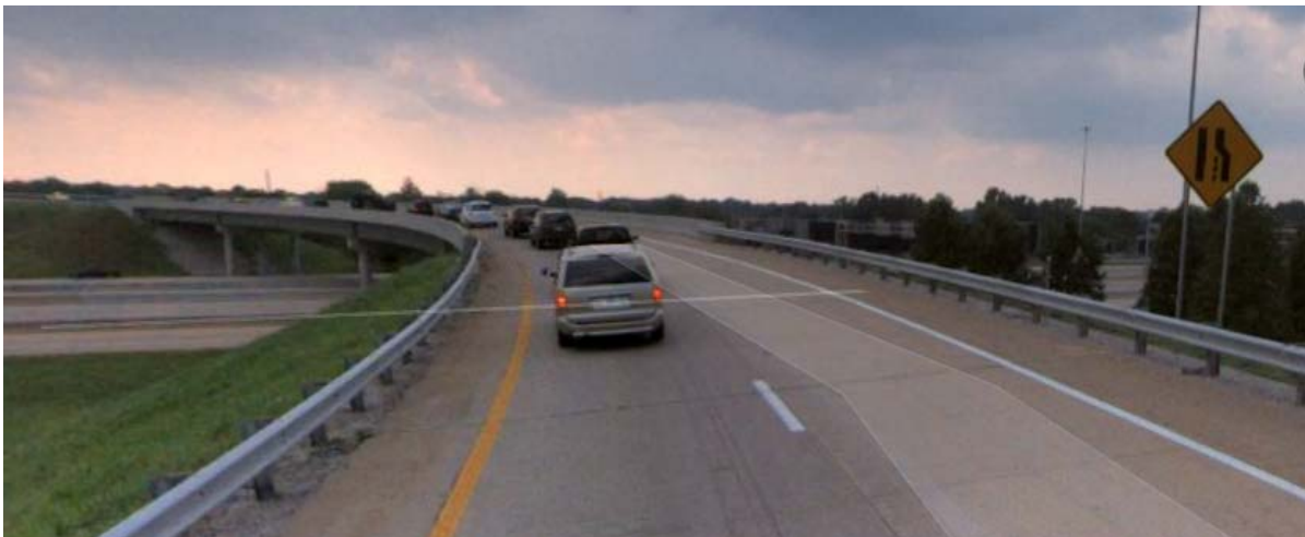
Existing right lane merge sign
